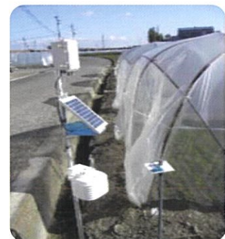
Monitoring ICT for simpler facilities
